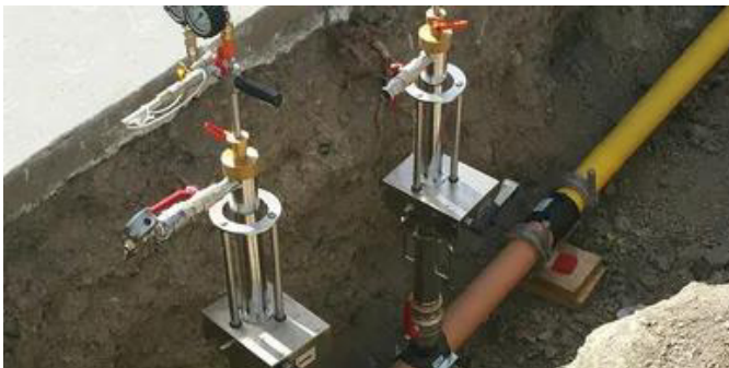
Kleiss stopper system controlling system flow on PE piping systems
