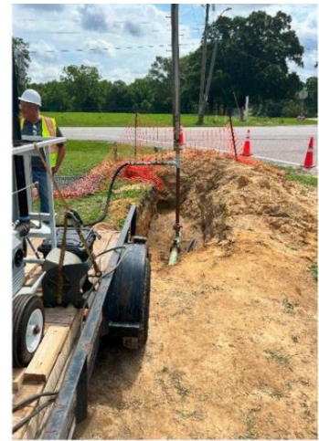
The vacuum purge system was attached to the new section of steel pipe - attached to the purge stack - and a vacuum was created in the new pipe down to approximately 14.5 psig
