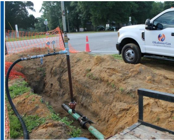
The vacuum purge system was attached to the new section of steel pipe - attached to the purge stack - and a vacuum was created in the new pipe down to approximately 14.5 psig
