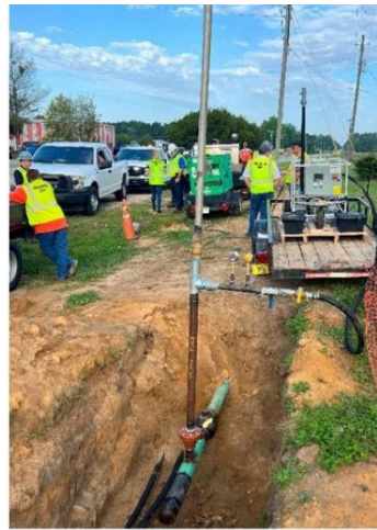
The vacuum purge system was attached to the new section of steel pipe - attached to the purge stack - and a vacuum was created in the new pipe down to approximately 14.5 psig
