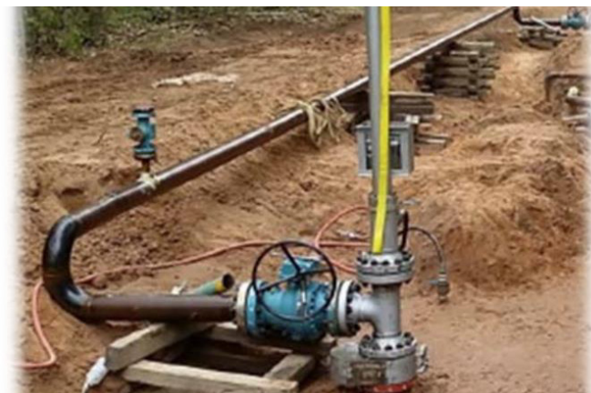
A below-ground pipeline section that has been isolated using stopples and an above-ground bypass line to avoid service interruption to customers
