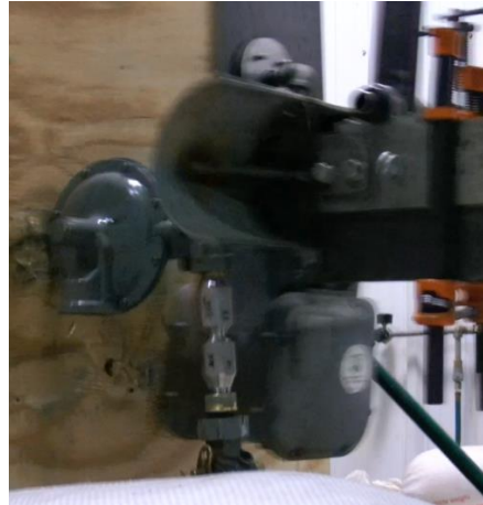
Figure 17: Head On Impact of Utility 8 Meter Set with Breakaway and Regulator Aimed at Wall
