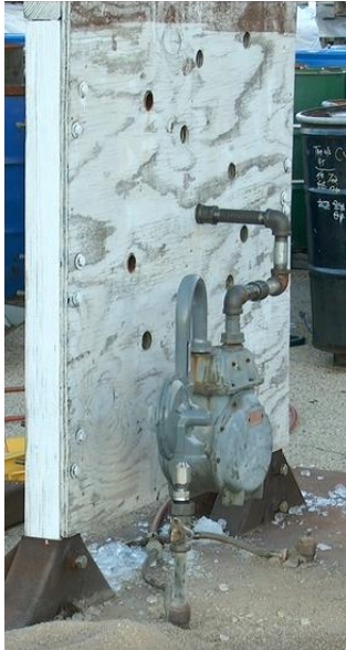
Figure 30: Drop Testing Setup of Utility 1 Meter Set with Breakaway
