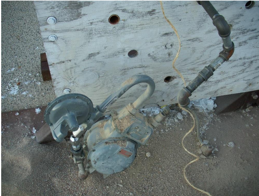
Figure 83: Utility 1 Meter Set with Breakaway After First Drop Test
