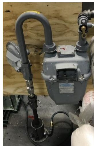
Figure 19: Utility 7 Meter Set (Without Connector Bar)
