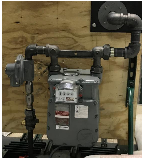
Figure 77: Utility 6 30 Lite Meter Set with Breakaway and Meter
