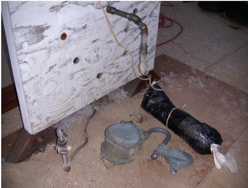
Figure 86: Utility 1 Meter Set with Breakaway After Second Drop Test
