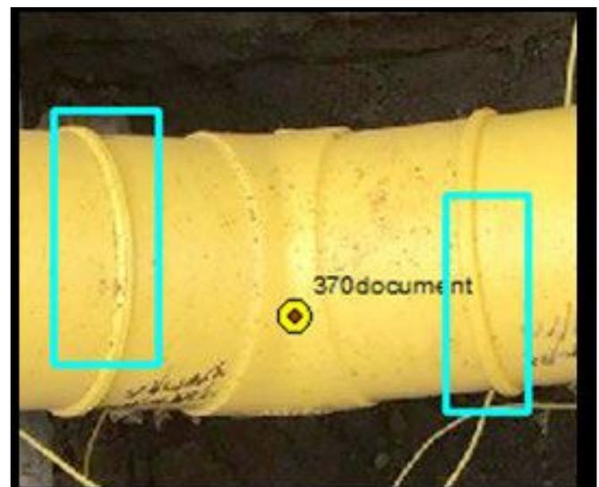
Multiple butt fusions being detected and extracted to GIS features from a single image.
