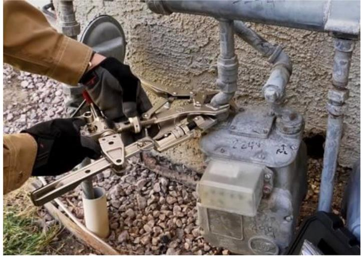
creating downstream gas leaks on customer piping due to the excessive stress and strain created from pipe-wrenching activities required to un-seize these fittings. This tool will improve employee and customer safety along with reducing time required to repair customer piping leaks created by during routine meter changes and removals.
