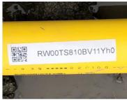
The objective of this project is to improve upon data-collection techniques used for tracking and traceability. By automating the data-collection process through digital-scanning techniques, field crews can remain safe outside of the trench and allow the scanner to capture the natural gas assets.
