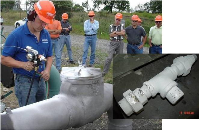
**Researchers investigated a flame powder system, which has been shown to provide coatings strong enough to withstand hammering (inset).**
